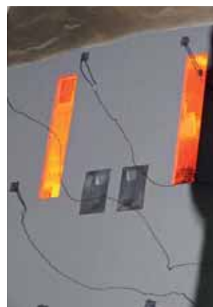
Panels of swing door following 120-minute fire test
